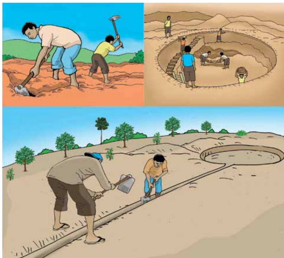
Figure 28. Rainwater reservoir under construction
