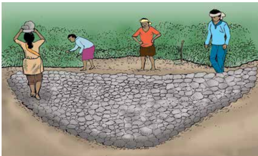
Figure 18. Loose stone check dam
