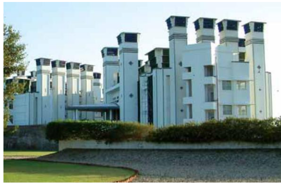
Figure 9. Passive Downdraught Evaporative Cooling in Torrent Research Centre, Ahmedabad.
