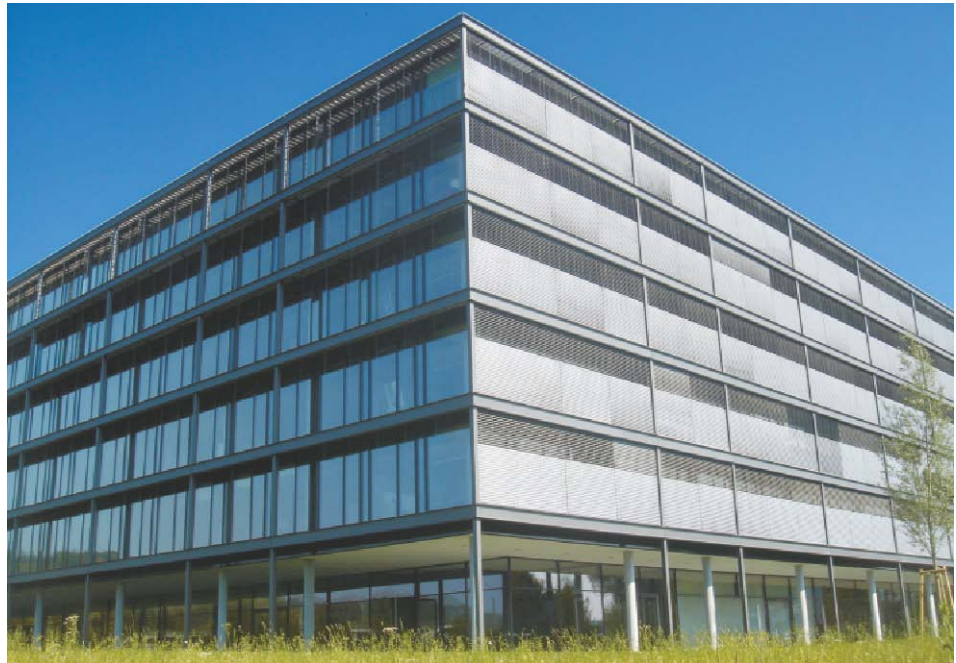
Fig. D3.10 View of the façade, shaded and sunny side
