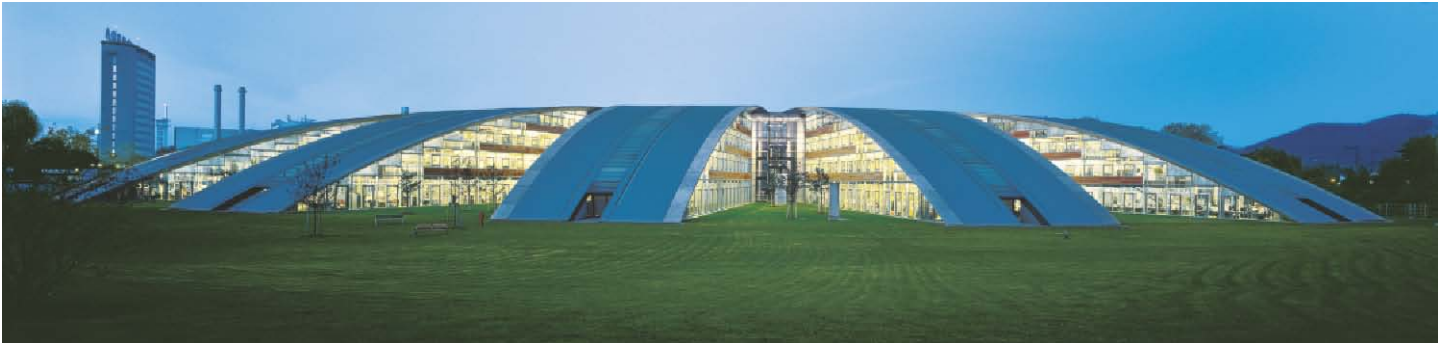
Fig. C1.54 The Burda Media Park in Offenburg, Germany. Architects: Ingenhoven Architekten, Duesseldorf
