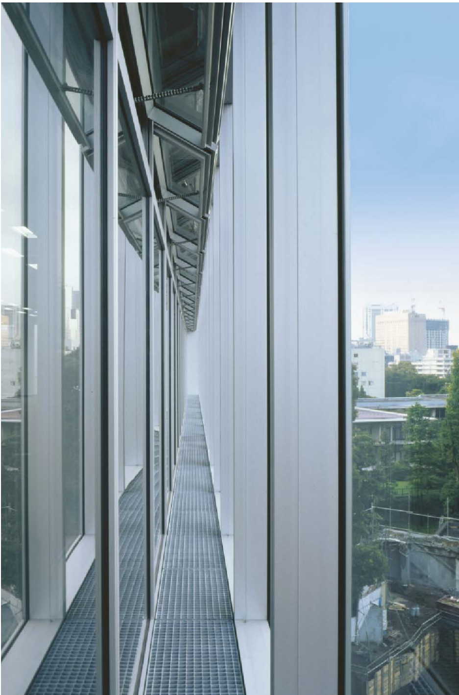
Fig. C1.74 Interior view of the double-skin façade of the Sekisui Building
