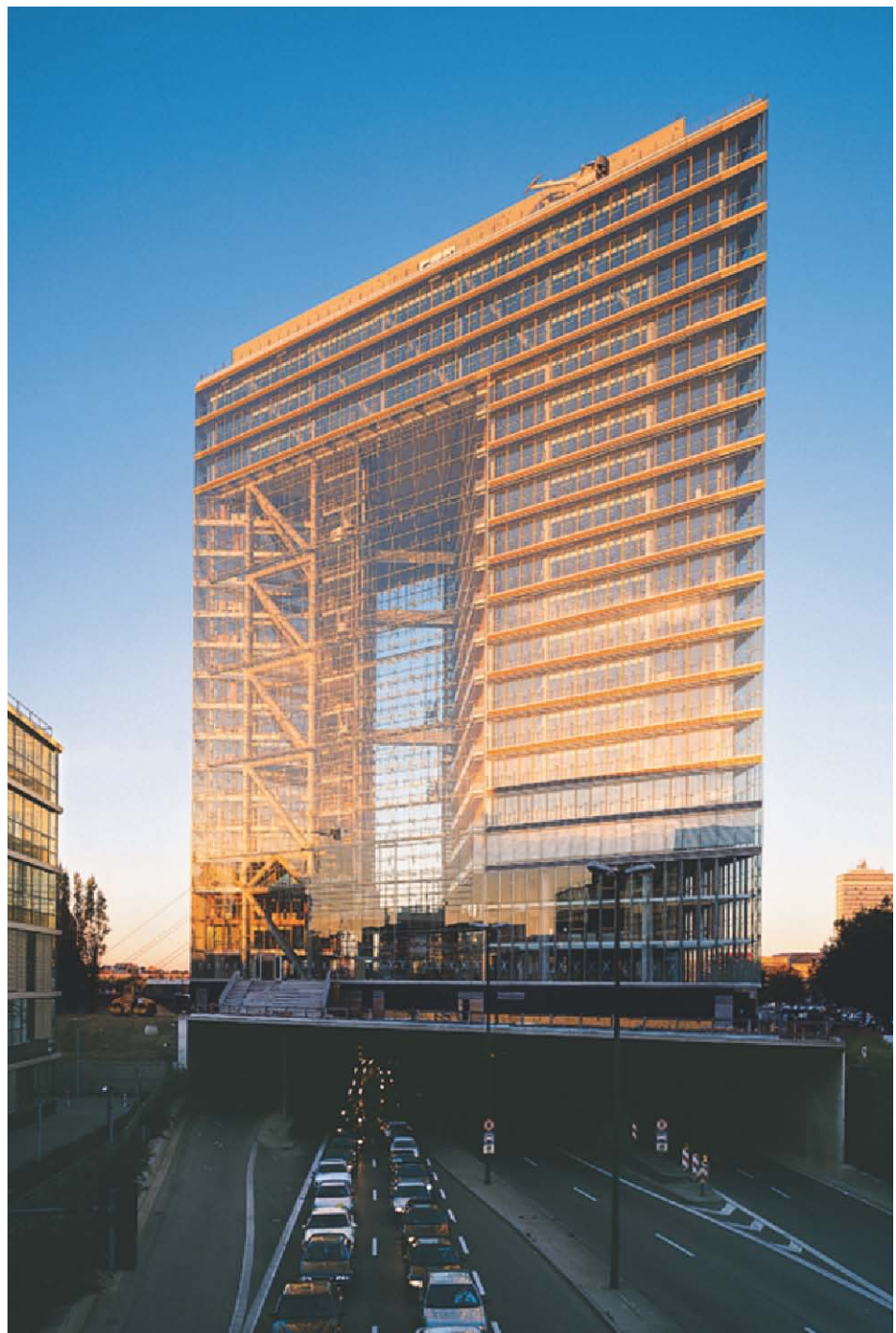
Fig. C1.67 Duesseldorf City Gate. Architects: Petzinka Pink Technologische Architektur®, Duesseldorf
