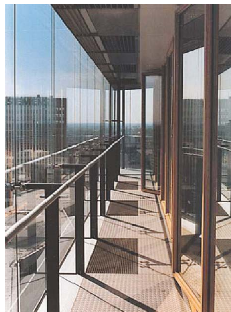
Fig. C1.68 View of double-skin Façade of Duesseldorf City Gate
