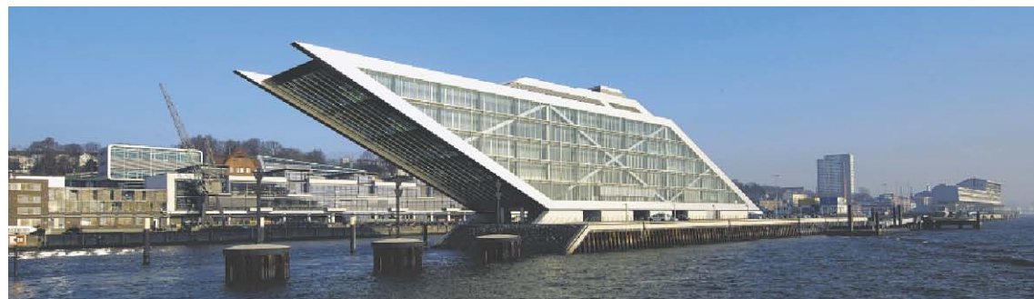
Fig. D1.1 Dockland Office Building, Hamburg/Germany
