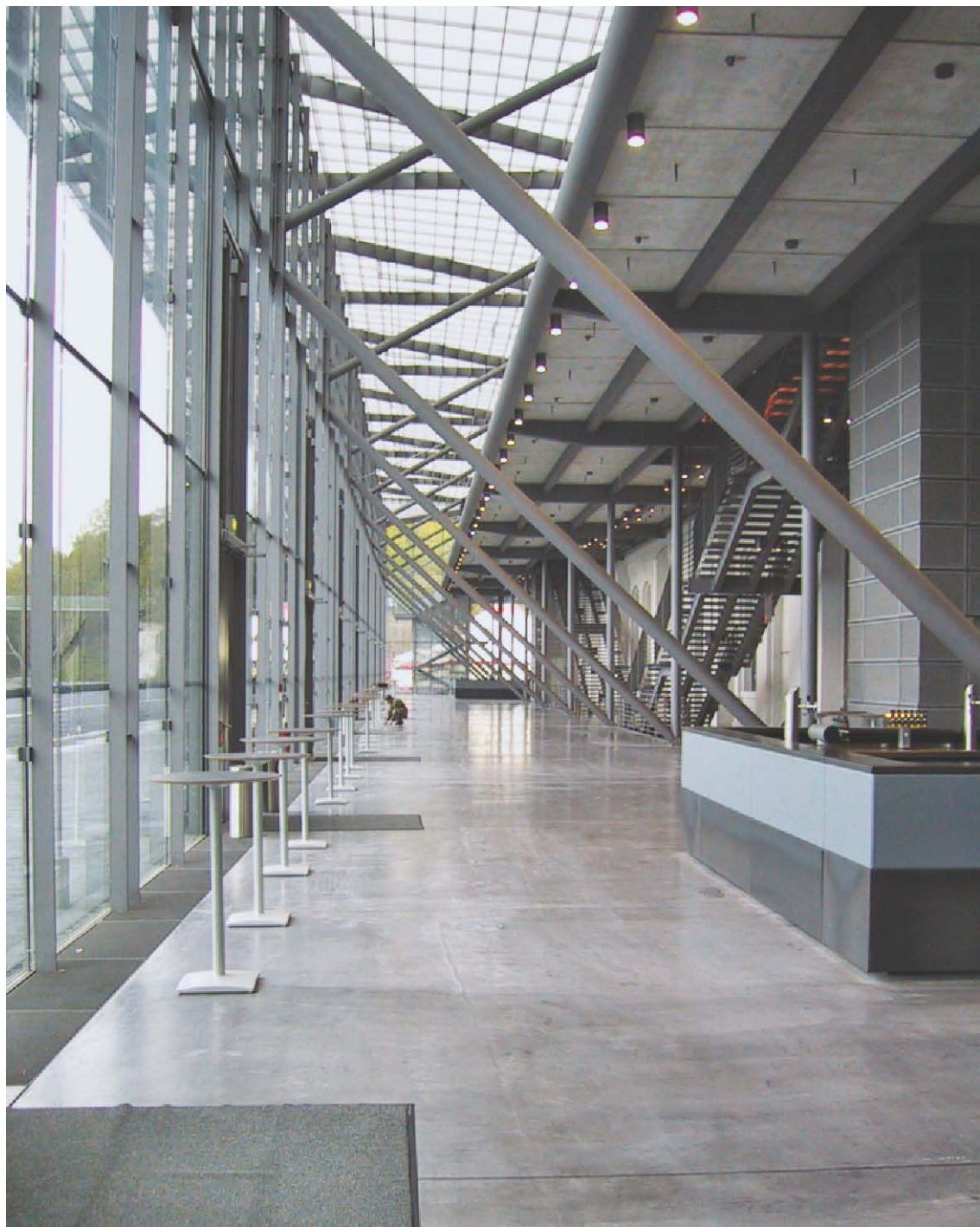
Fig. C1.15 Bochum Century Hall after revitalisation. Architects: Petzinka Pink Technologische Architektur®, Duesseldorf
