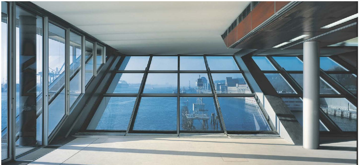
Fig. D1.2 View from the tilted façade onto the river Elbe
