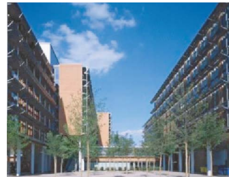
Fig. D2.3 View between the two new building sectors
