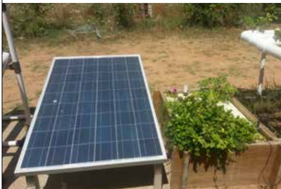
FIGURE 9.10 Photovoltaic cells used to power a water pump
