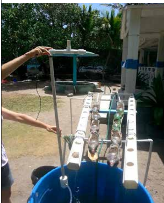
FIGURE 4.42 Simple water airlift
